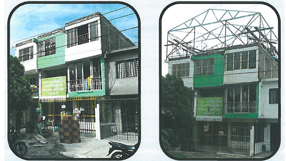
Above, a new concrete deck has been poured to create a base to build on & below, a steel structure to support walls and a new roof to provide the necessary accommodation
