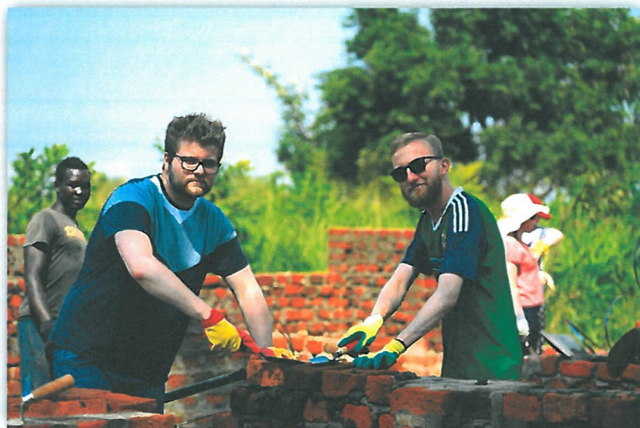
Jordan (left) and Harry (right) helping to build accommodation for teachers
